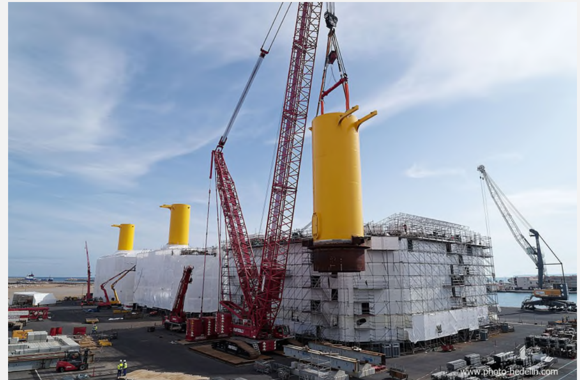
Eolmed: Assembly of final transition piece at the yard
